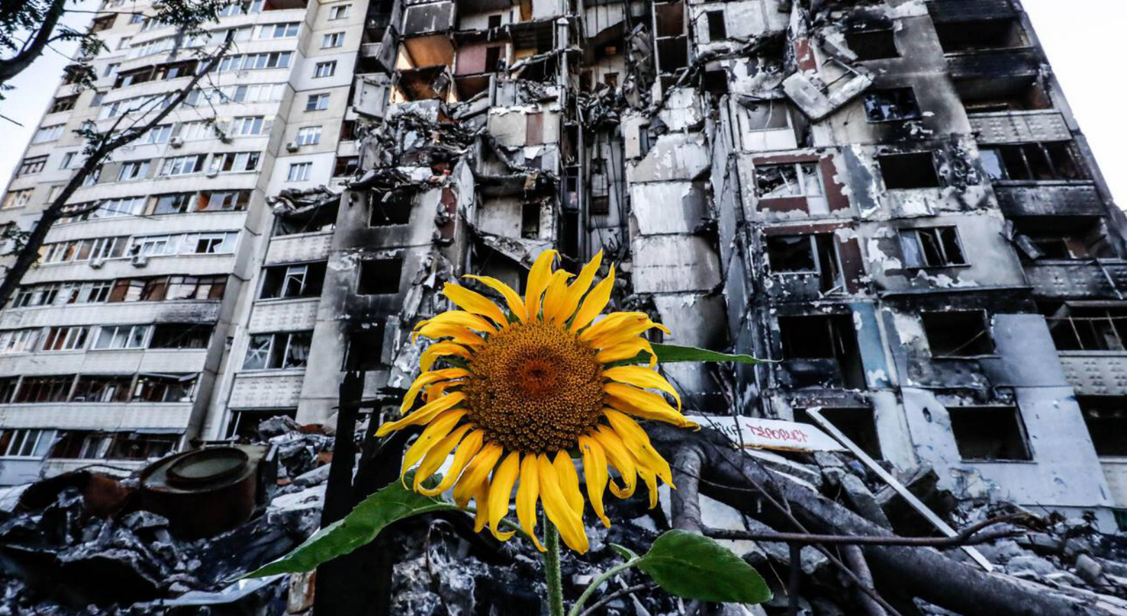
Kharkiv, Ukraine. 7th Aug, 2022. A sunflower is seen among the debris of a heavily damaged apartment building following a Russian air strike on a Kharkiv residential area. Credit: Daniel Ceng Shou-Yi / ZUMA Press Wire / Alamy Stock Photo
