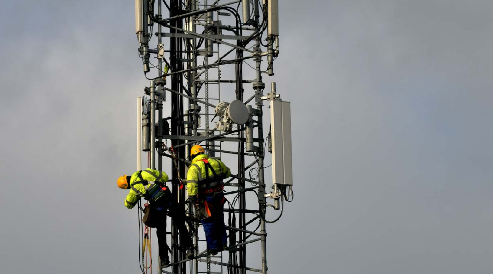
Photo: Telecommunications technicians repair a phone network antenna in Dublin, Ireland. (Jan 16, 2009). Credit: Douglas O'Connor.
