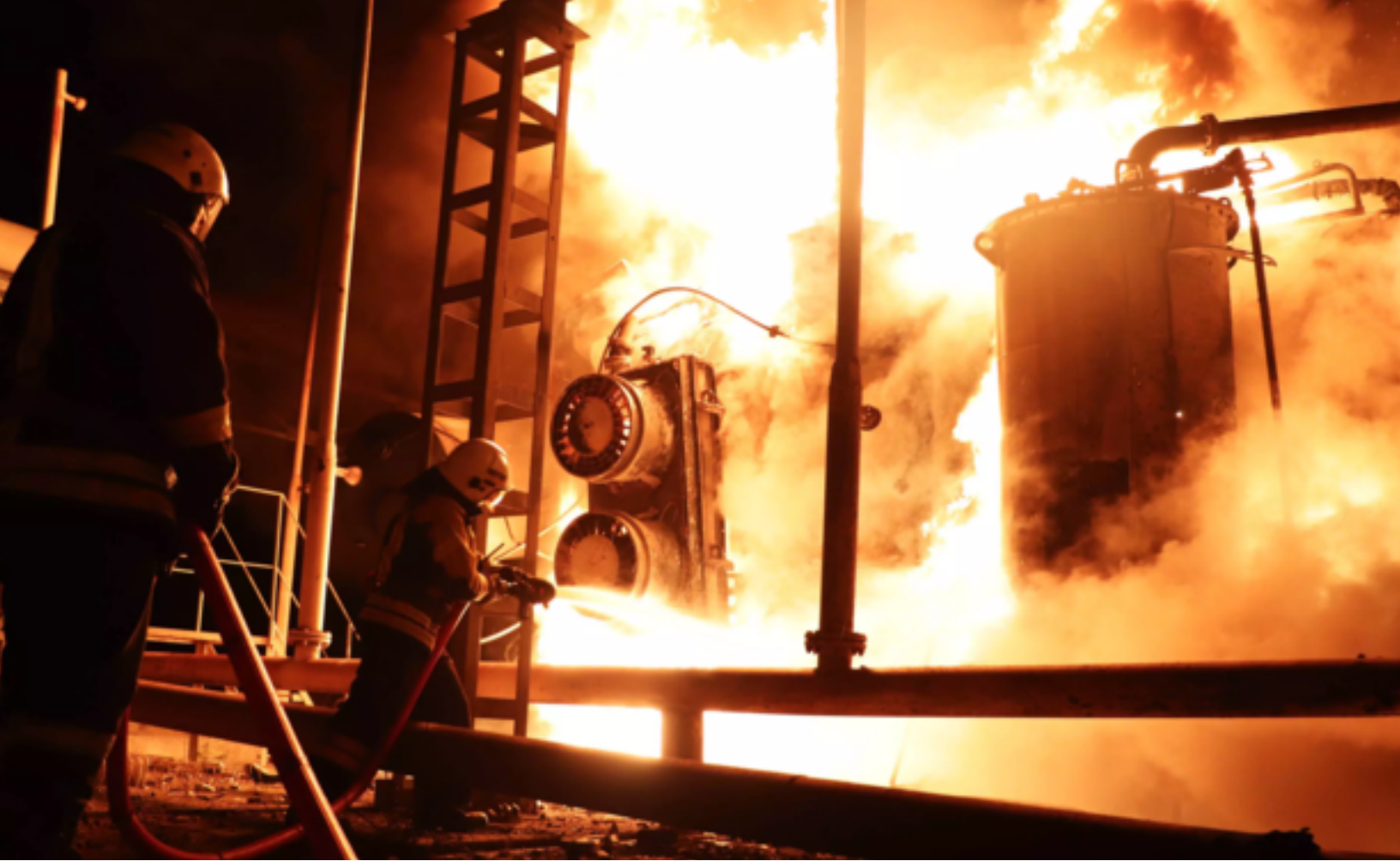
Photo: Energy infrastructure destroyed by Russian drone strike, October 27th, 2022. Credit: State Emergency Service of Ukraine.
